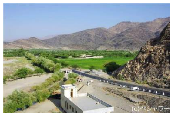
After project completion
